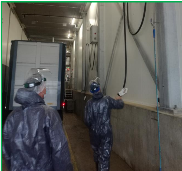
Make sure cross-ventilated trucks can connect to a power supply, so their fans always work, as seen at Westfort slaughterhouse in IJsselstein (NL).
