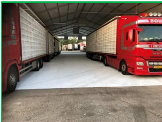
Whitewashed floor and white roof to reflect sunlight at VION Boxel and Remkes in Epe.
