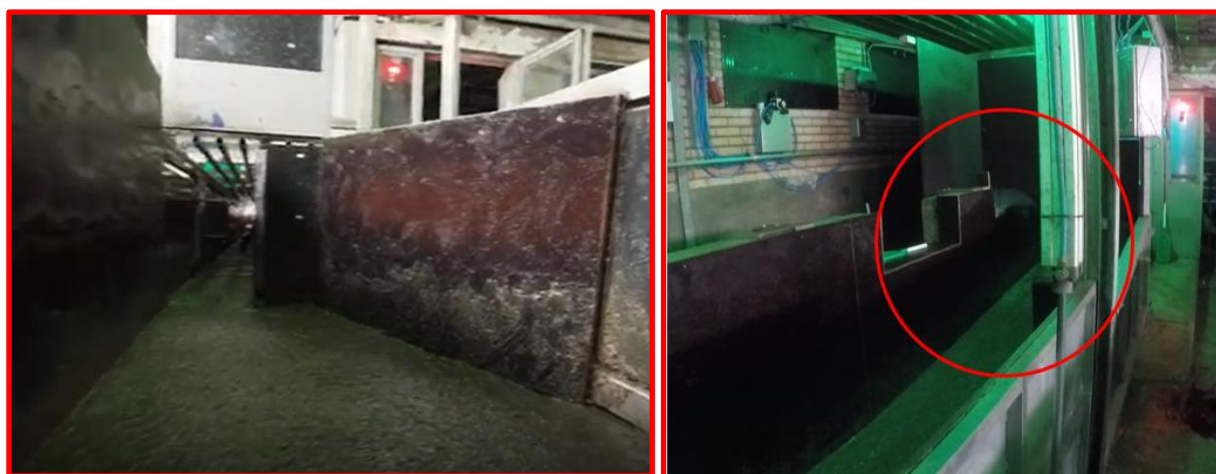
The entrances to these single file raceways are not well lit – pigs will be scared to enter. Add lamps.
