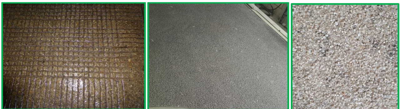
Non-slip floor unloading dock
