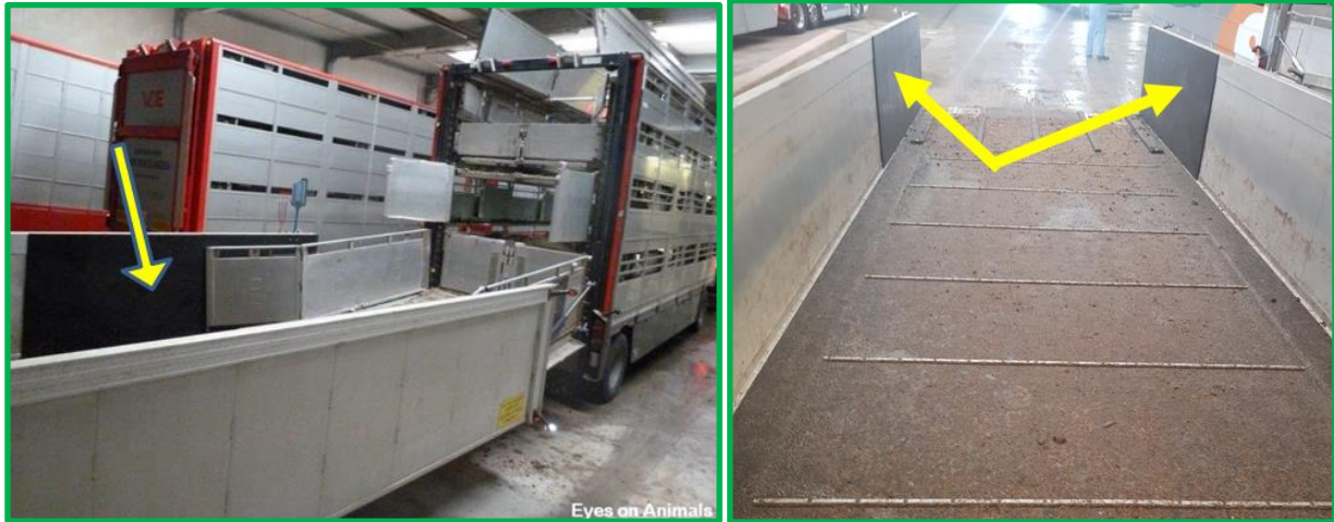
Rubber panels to reduce noise (from metal to metal contact) at Compaxo pig slaughterhouse in Zevenaar (NL)
