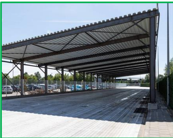
Whitewashed floor and white roof to reflect sunlight at VION Boxel and Remkes in Epe.
