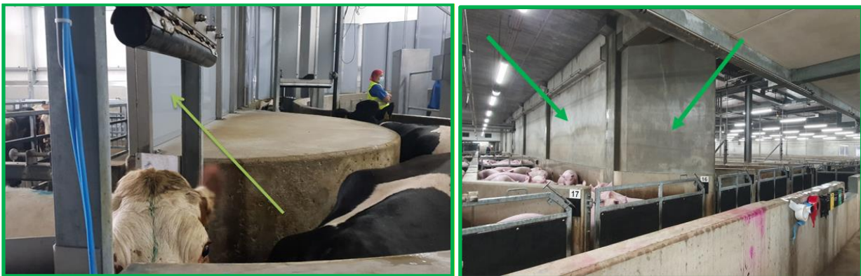
By installing a noise reduction wall between the lairage and the rest of the slaughterhouse, the noise level in the lairage at Ameco cattle slaughterhouse has been significantly reduced (left photo). At Compaxo, a noise reduction wall was installed to prevent echoes and noise from spreading (right photo) through the lairage.
