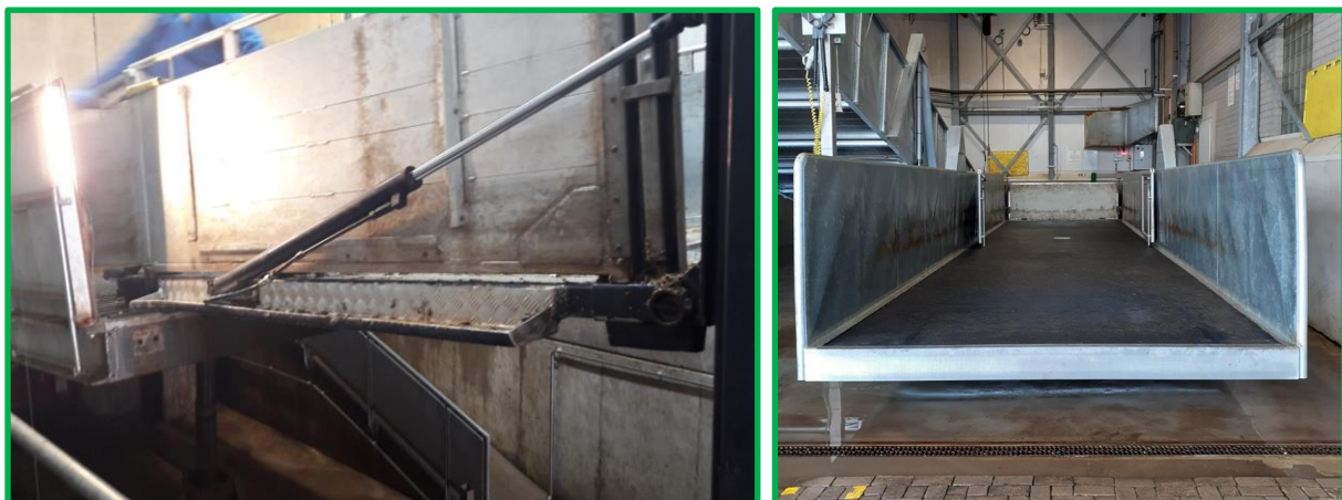
A loading platform that can be set at different heights so the gradient is minimal
