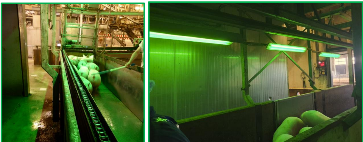
Green lighting installed at Tönnies (DL) and Van Rooi (NL) to reduce the creations of shadows
