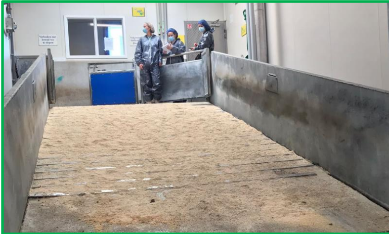
At Westfort slaughterhouse in Gorinchem (NL) (when it was still open), they would sprinkle sawdust on the loading docks to reduce sharp contrast and improve grip.
