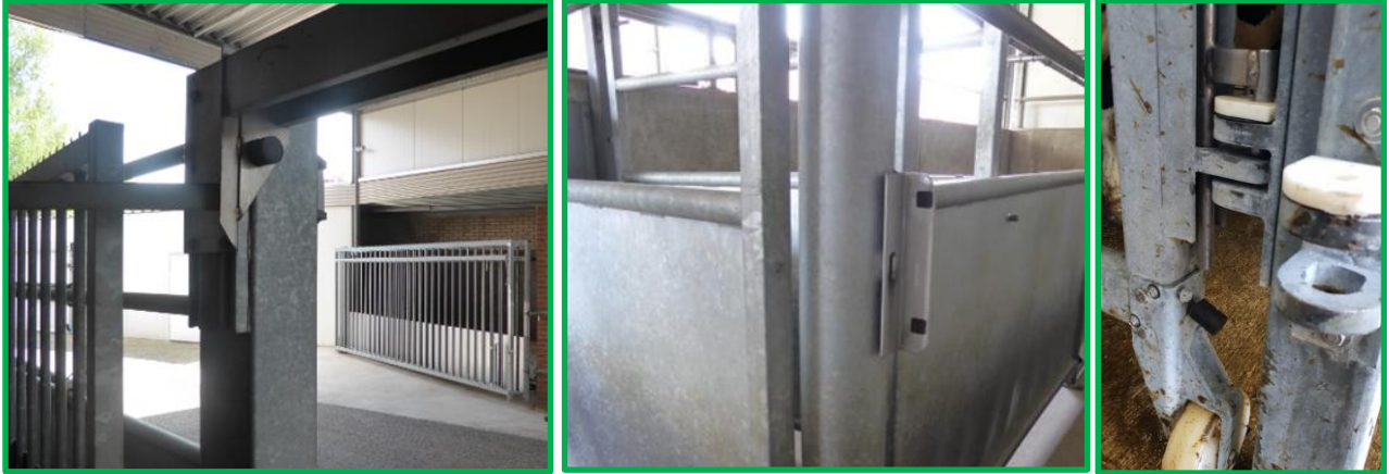
Mounting rubber helps in reducing loud bangs when gates are closed
