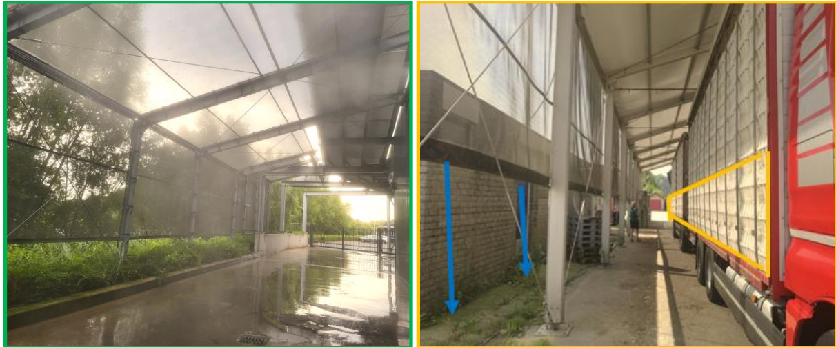
Left: sufficient lateral shade-netting at Westfort slaughterhouse in IJsselstein. Right: the shade-net at this slaughterhouse cannot be closed fully down to the ground (see blue arrows), the lower crates (see orange markings) are therefore still exposed to the sun.
