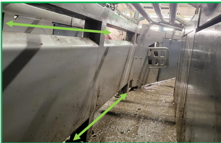
At Compaxo, the wall between the two single-file raceways was opened at the bottom and top so pigs can see each other and have the feeling that they are walking still side by side, which feels safer for them.
