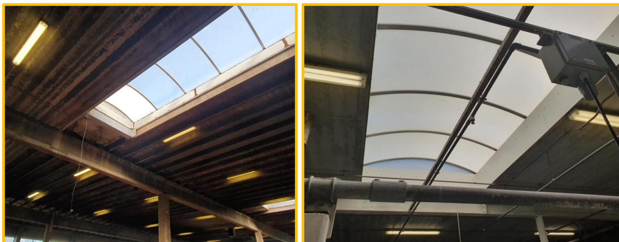
Skylights can cause temperatures to rise very quickly
