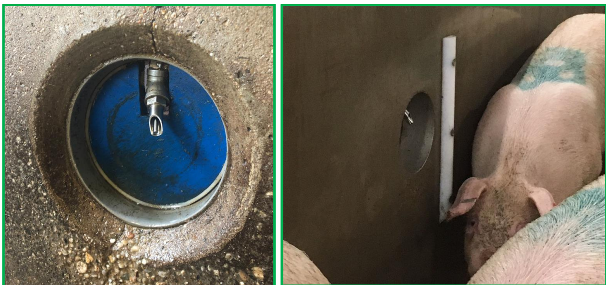
Most ideal are water-nipples integrated directly into the wall, so they do not protrude
