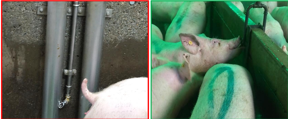
Left photo: Nipple too close to pipe rendering it inaccessible. Right photo: Correct nipple.
