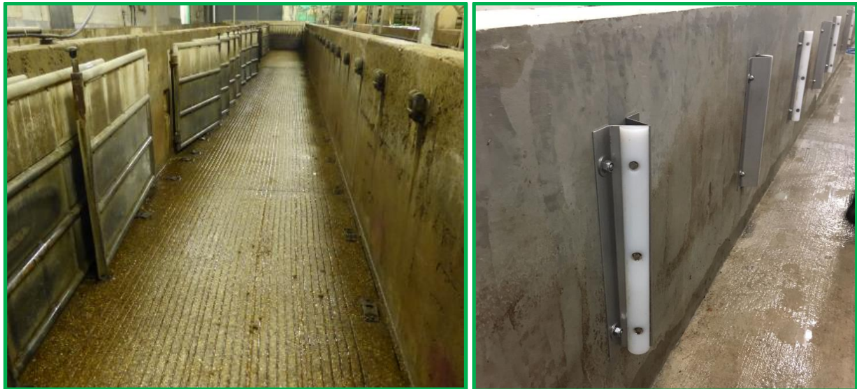
Lairages at Tönnies (DE) and Westfort (NL) with partitions to reduce the mixing of pigs from different social groups
