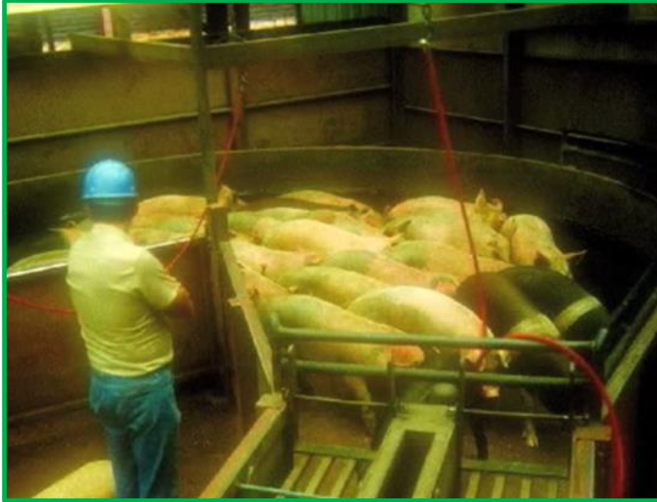
Round crowdpen leading to two single file raceways (with a see-through divider in-between) will reduce stress as pigs can still walk side by side, which feels safer for them. © T. Grandin
