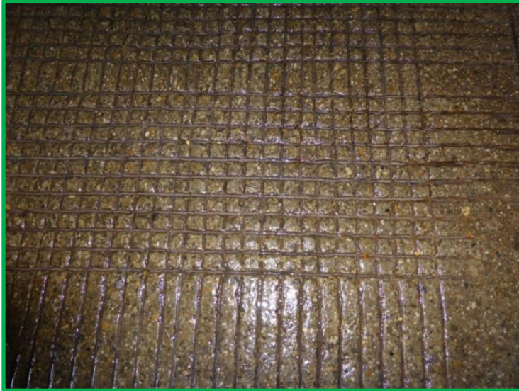
Create non-slip flooring to prevent the pigs from slipping
