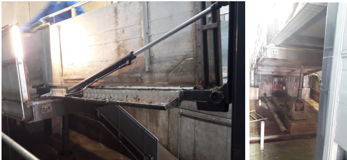
A loading platform that can be set at different heights (hydraulic)
