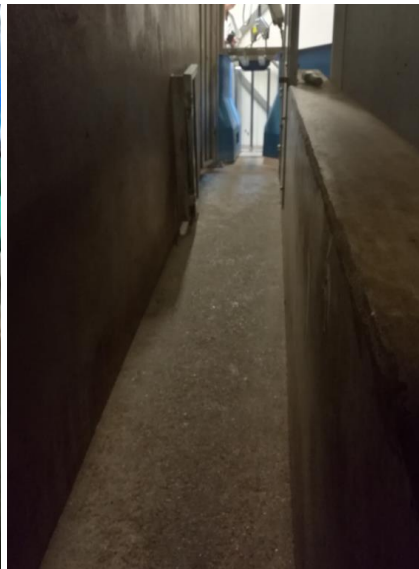
A raceway with a slope going upwards makes it difficult to move the pigs
