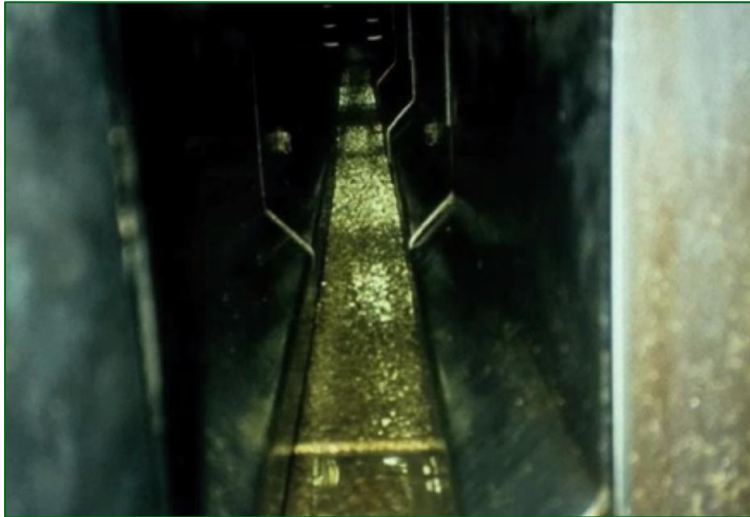
Due to the shadows and the reflections on the wet floor of this chute, pigs will balk. © T. Grandin
