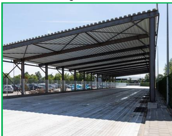
Whitewashed floor and roof to reflect sunlight at VION Boxtel
