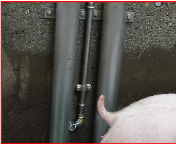
This nipple cannot be used easily as it is placed too closely to the pipe
