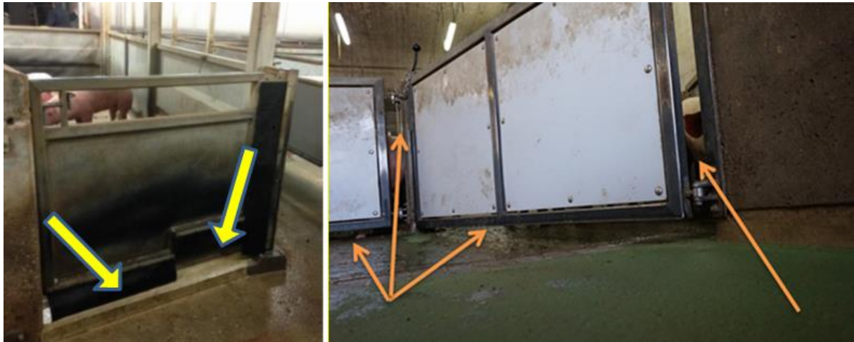
Anti-draft curtains at Westfort pig slaughterhouse in the Netherlands (left photo) and open gaps in the side walls of the pens cause unwanted drafts (right photo).
