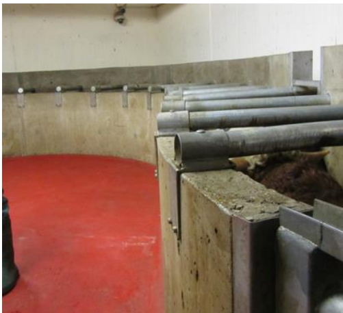
Raceway with closed walls and anti-jumping fencing
