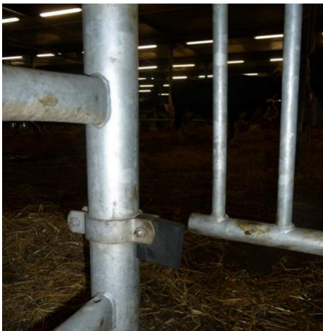
Placing of rubber nobs to reduce sound when opening and closing the gate
