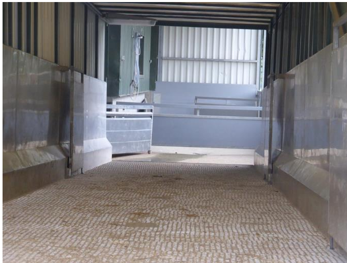
Ensure the sidewalls of the loading ramp are adequately high and solid
