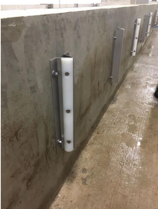
Partitions with sound reducing materials (plastic and rubber).
