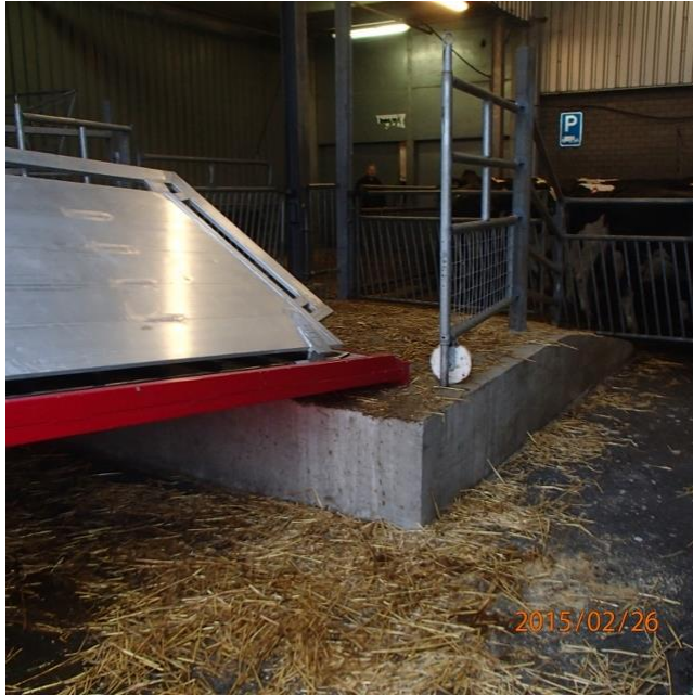
Loading platform at the livestock market in Leewarden (angle of the tailgate is reduced).
