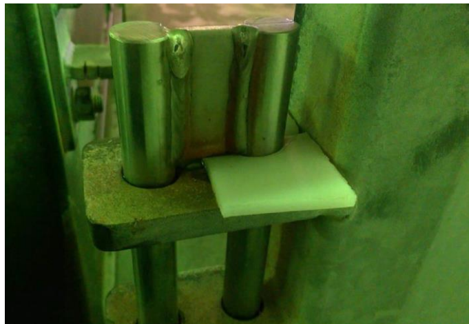
Placing of rubber nobs to reduce sound when opening and closing the gate
