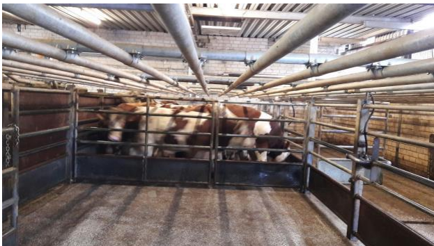
Anti-mounting fence "ceiling" above the lairage pens
