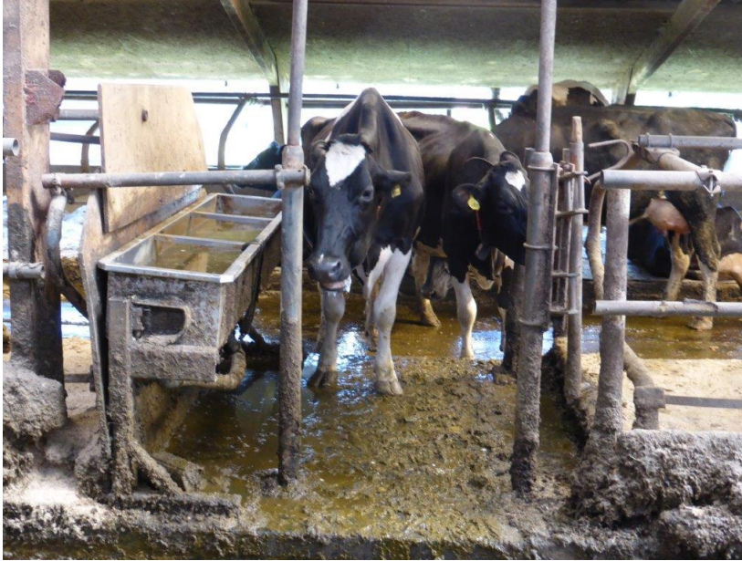
Figure 30. Queues due to misplaced drinking troughs, as the animals cannot pass each other in the narrow passageway. In addition, the passageway is very dirty and slippery and has a stair, which increases the risk for accidents.
